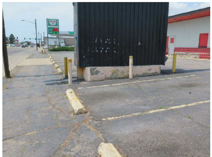
A dilapidated sign on deteriorating asphalt, serving as the public sidewalk
