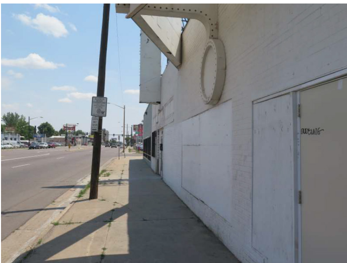
Boarded windows and doors
